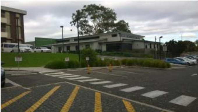
1. Huntington's Disease Unit – built 2012 and in good condition
