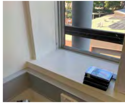
Smooth window sills and clean junctions
