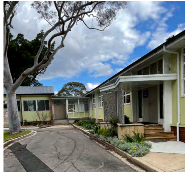
Image: 1-2 storey FASS laboratories at east of site
