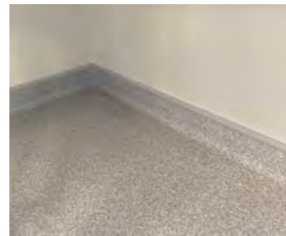
Coved skirting are generally smooth and well sealed to walls
