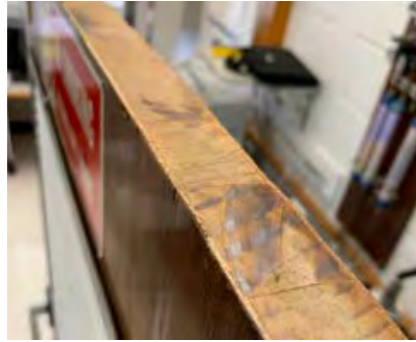
Typically tops of all timber doors are not sealed. Assume the same applies to bottom edge of doors.
