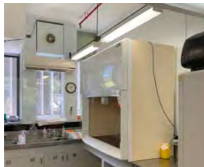
Positioning of fume cupboard may not be compliant, in relation to a/c split unit blowing air towards fume cupboard sash.
