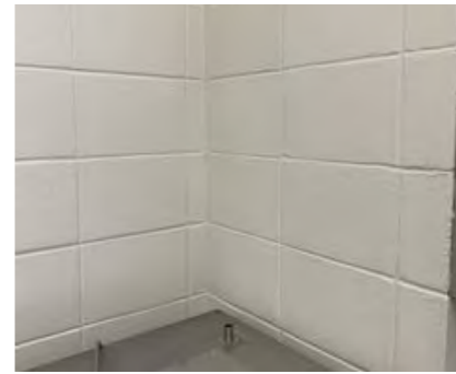
Painted blockwork wall with expressed joints in a number of rooms
