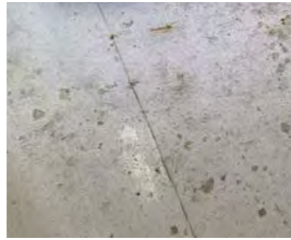
Stained vinyl flooring with deteriorated welded joints which are failing.
