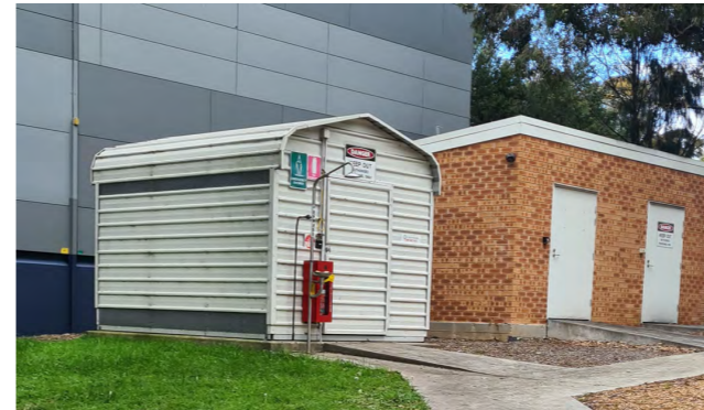
Image: dangerous goods store
