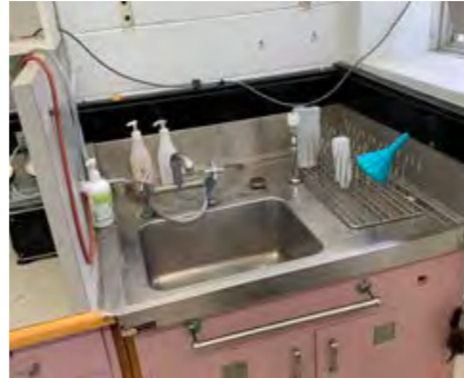
Timber joinery throughout. Walls not smooth or easily cleanable.
