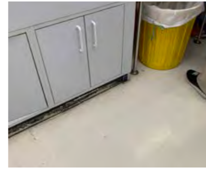
Generally timber joinery throughout labs.
