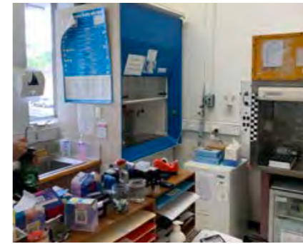
Positioning of Fume cupboard is non-compliant. Needs to be min 300mm off the wall. Access to it is also congested.
