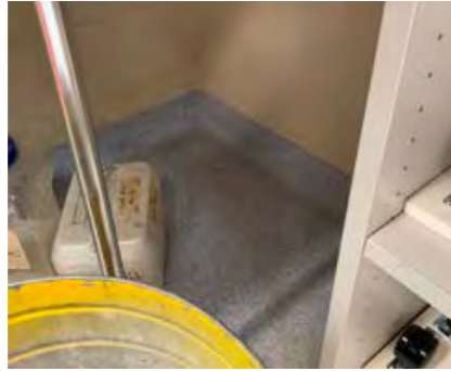
Room G32 - Upgraded vinyl flooring with coved skirting.
