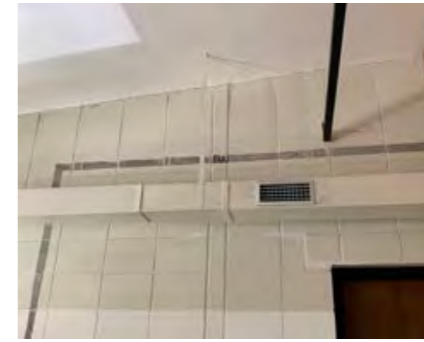
Blockwork with exposed mortar joints
