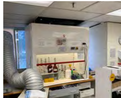
Ceiling cavity exposed to room. Possible contamination risks.
