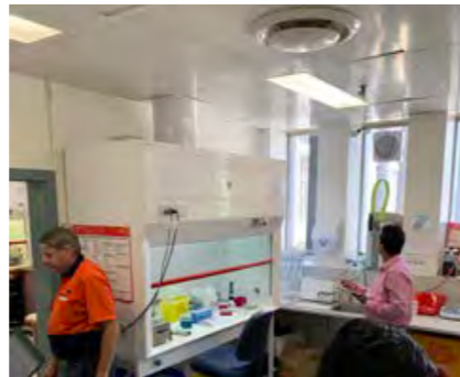
Fume cupboard location maybe non-compliant. Too close to door opening and air register.
