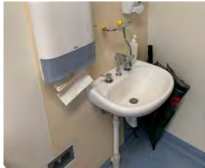
G22 lab has had some refurbishment. Compliant eyewash station and vinyl flooring with coved skirting.
