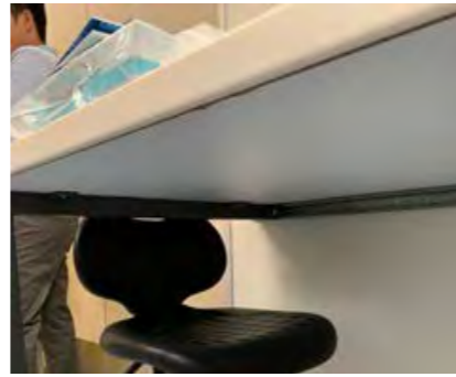
G22 lab - Seamless benchtops with sealed undersides. Some exposed timber at drip edge needs to be sealed.
