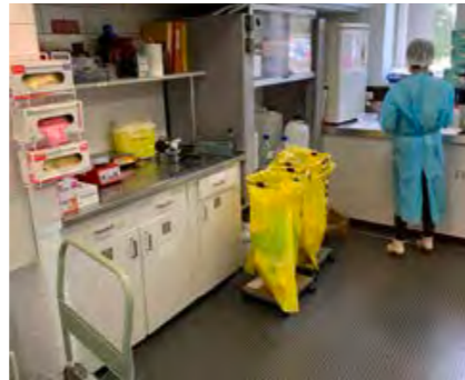
Mosaic tiled floor difficult to clean.
