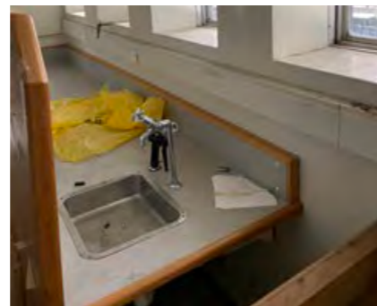
Fixed joinery with exposed timber
