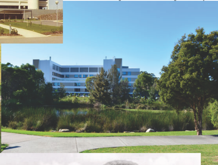
Figure 2. View of new Building D from Birunji Creek
