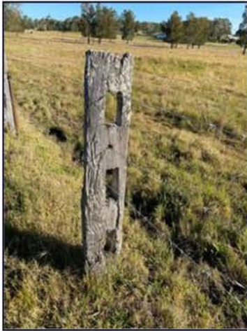
Photograph 8: A three rail fence post. View to south-west.
