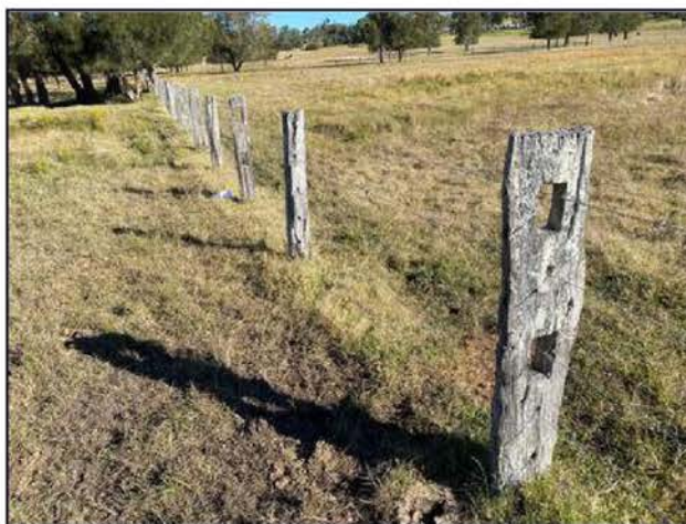
Photograph 7: Wooden fence posts along western border with evidence of former post and rail construction. View to south-west.
