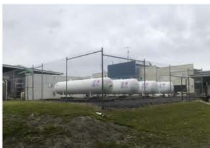
Figure 6: LPG storage vessels on site
