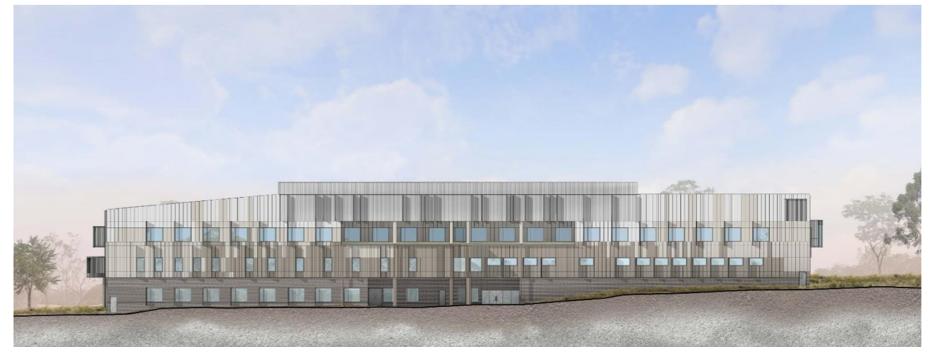
FIGURE 52 – SOUTHERN FAÇADE 'METAL' SKIN – SOUTH ELEVATION OF SOUTHERN WING
