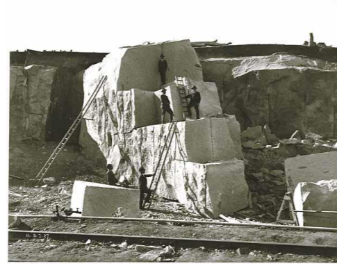
FIGURE 10: MORUYA GRANITE QUARRY - 1864 (RESOURCE: MORUYA GRANITE QUARRY - 1864- | WWW.ENGINEERSAUSTRALIA.ORG.AU)
