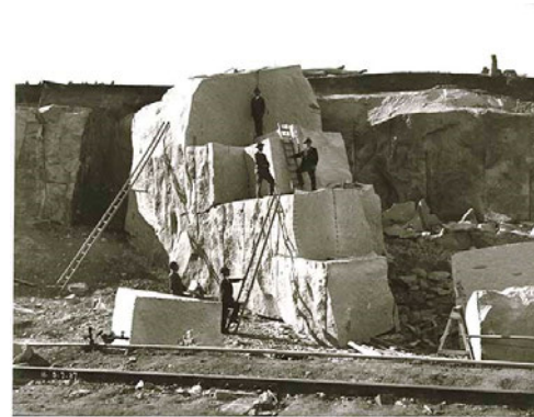
Figure 12: Moruya Granite Quarry - 1864 (Resource: Moruya Granite Quarry - 1864- | www.engineersaustralia.org.au )
