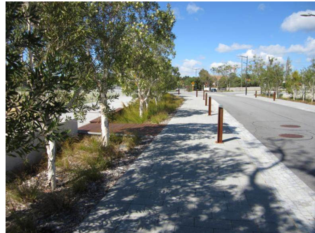
Figure 31: Attractive road and pedestrian corridors with integrated WSUD catchments (Source: https://www.water.wa.gov.au/urban-water/urban-development/urban-water-design/ )
